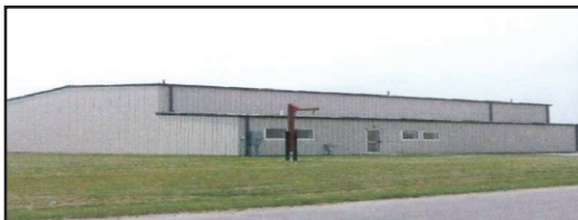
102 Crestview Drive Extension (Bldg. #10)
