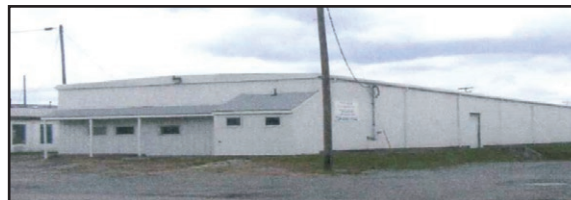
541 Fourth Street (Bldg. #5)
